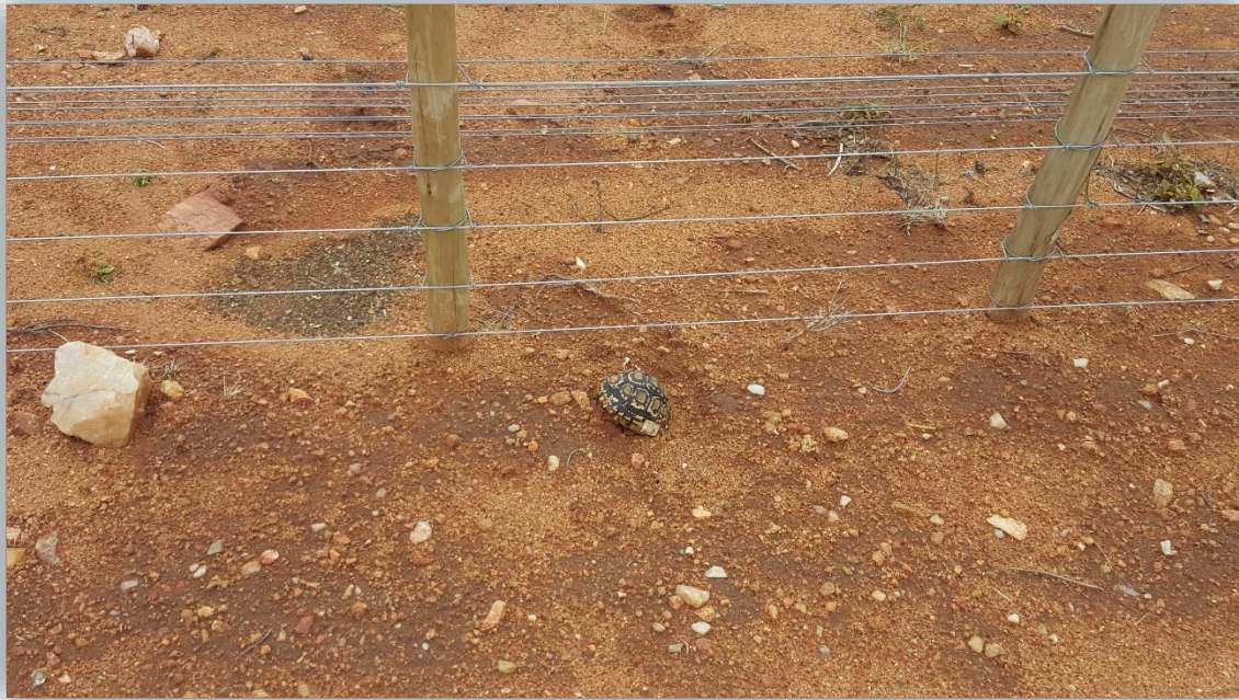
Figure 1: Unintended consequences of electric strands very low to the ground. Various invertebrate and vertebrate species electrocuted when trying to move underneath this fence at an intensive breeding facility in Limpopo Province.
